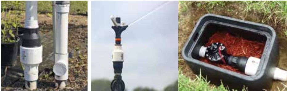
Always install downstream from all shut off valves.
