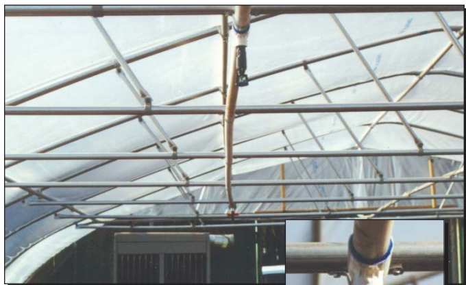
The i-mini-Wobbler® shown above with the Drain-Stop Valve, irrigates 36 mm plugs about 6 ft above the bench in a covered 32-ft quonset-style greenhouse.
