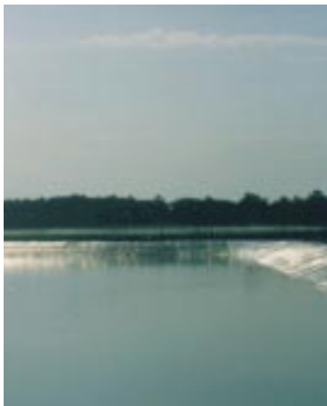
The holding pond capacity is 15.3 million gallons.
