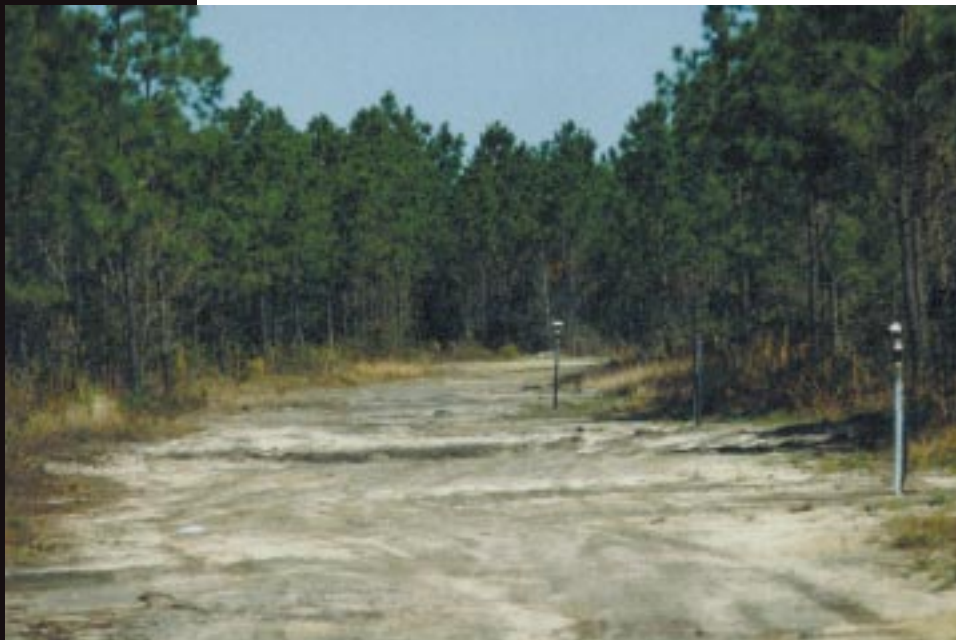
The land treatment spray fields use over 18,000 Senninger sprinklers at a spacing of 60 feet x 80 feet to cultivate pine trees and create an environment for wildlife.
